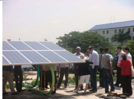
TCEP participants observing Photo Voltage Solar Cell at the Services and Environmental Quality Development Center, Nonthaburi
